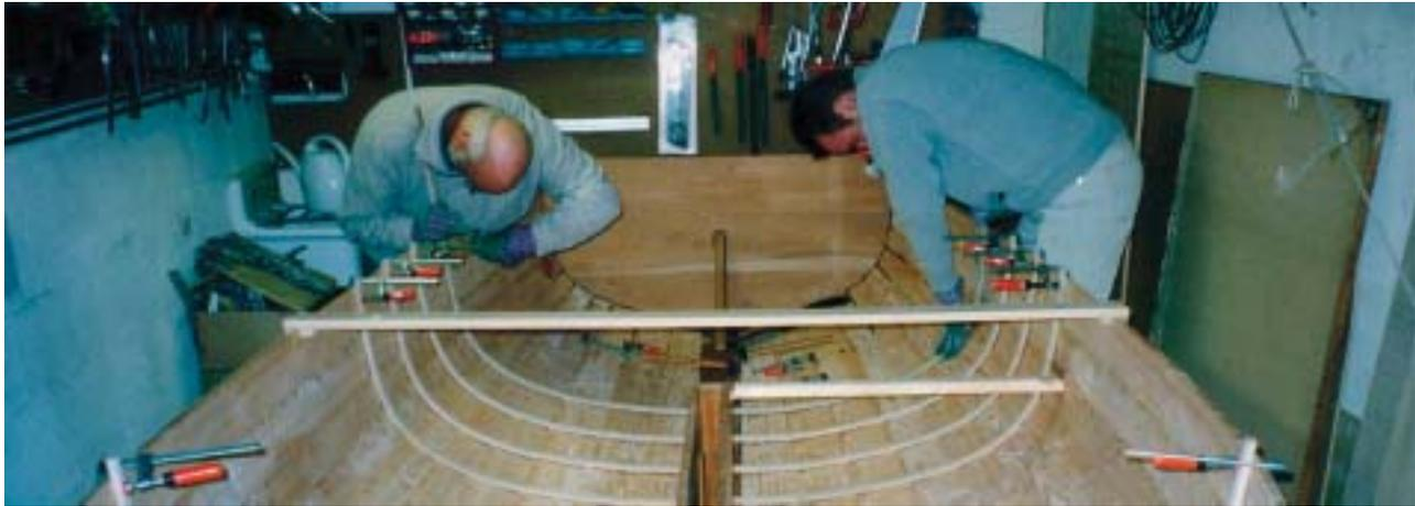
**Above:** The timbers – frames – were made from green oak which steams very well. My son and I worked as a team, pushing the longest frames into place first so that any breakages might still be able to be used in the bows or beside the c/b case. We made sure of a snug fit at the turn of the bilge. After cooling overnight, the frames were numbered and then removed to allow them – and the inside of the hull – to be sanded down and then given three coats of the French le Tonkinois varnish.
